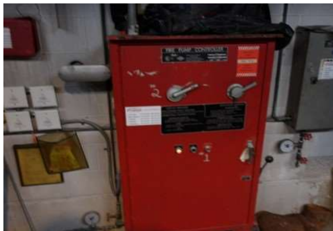
Fire pump controller
