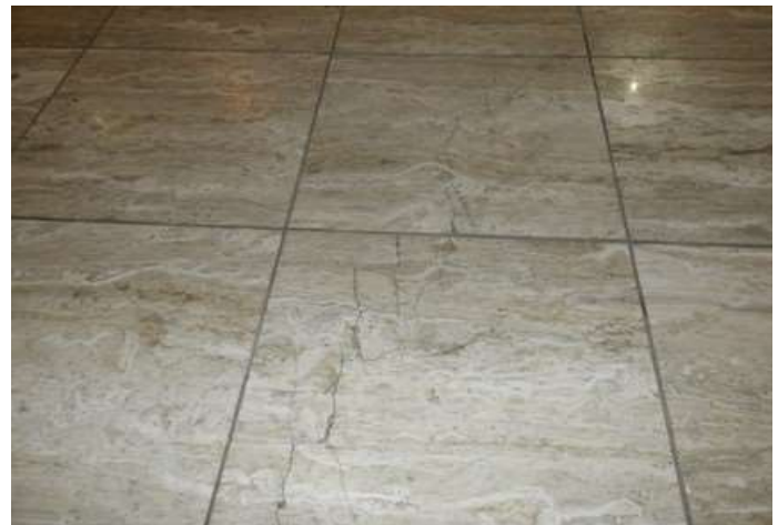
Cracked floor tile
