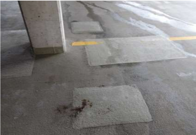
Previous concrete patches
