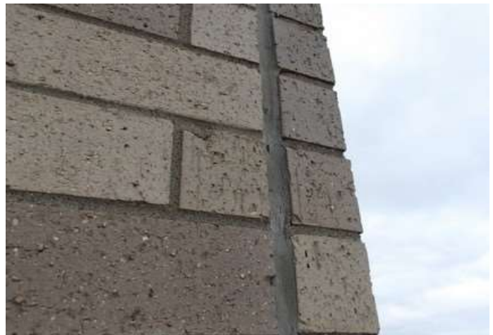
Control joint sealant detail
