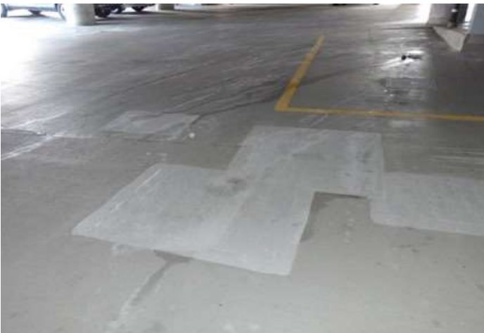
Previous concrete patches
