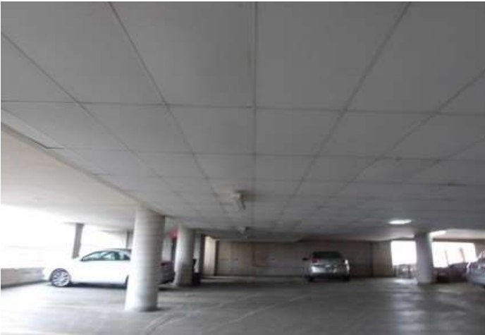
Dropped ceiling tile and grid system
