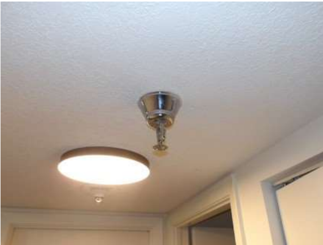
Sprinkler head in hallway
