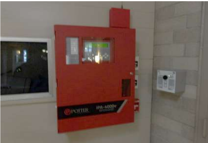
Fire alarm control panel
