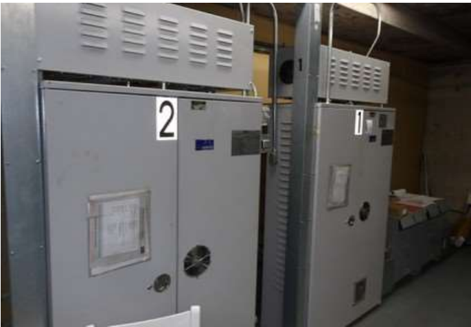
Elevator controls
