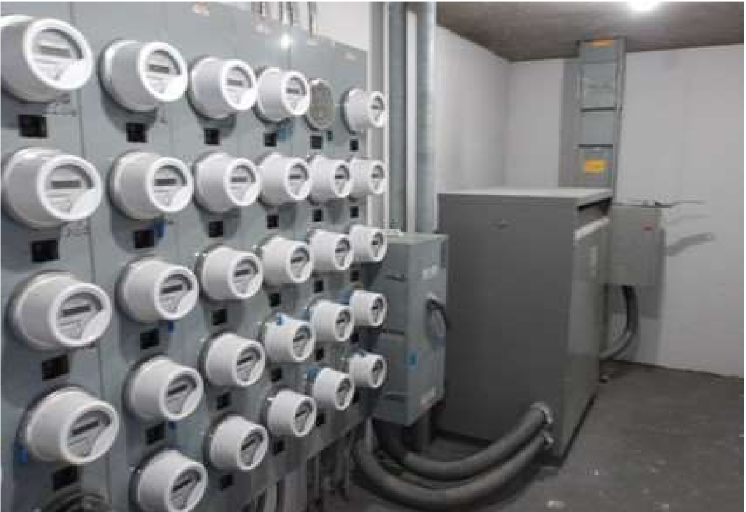
Typical meter room with transformer
