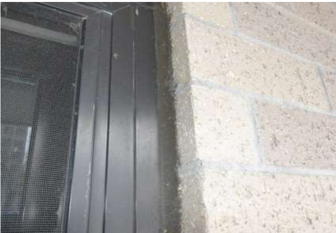
Window sealant detail
