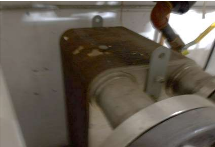
Building heating plate heat exchanger
