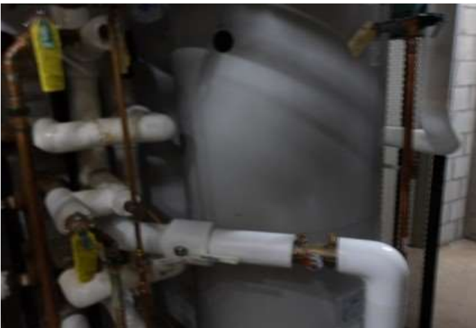
Insulated storage tank
