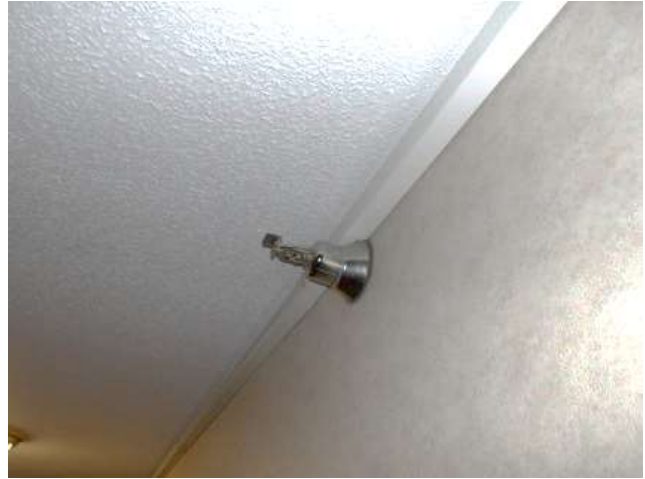
Fire suppression sprinkler head
