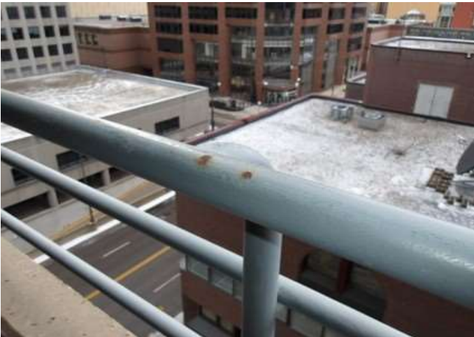
Rust at metal railing
