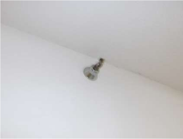
Fire suppression sprinkler head
