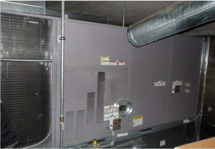
Packaged heating and cooling unit
