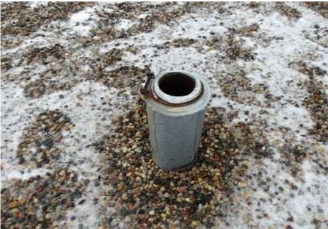
Vent pipe penetration through roof
