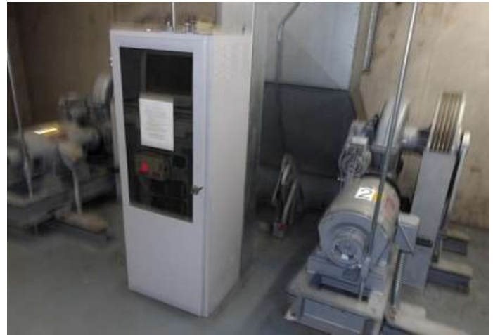
Elevator hoist and controls
