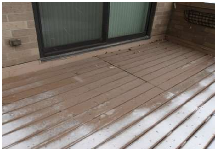
Wood decking over roof membrane
