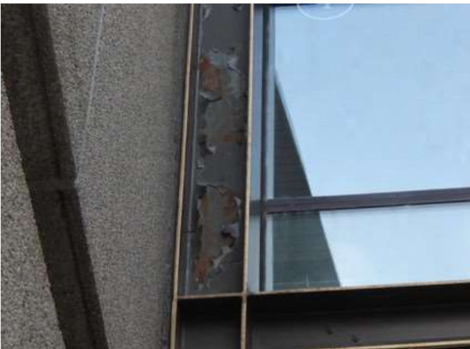
Rust and peeling paint
