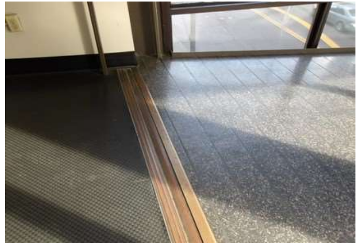
Expansion joint between skyway and building
