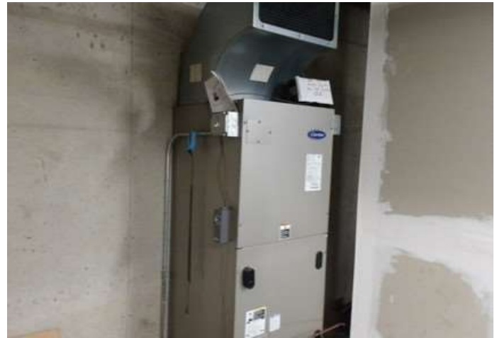
Elevator control room air handling unit
