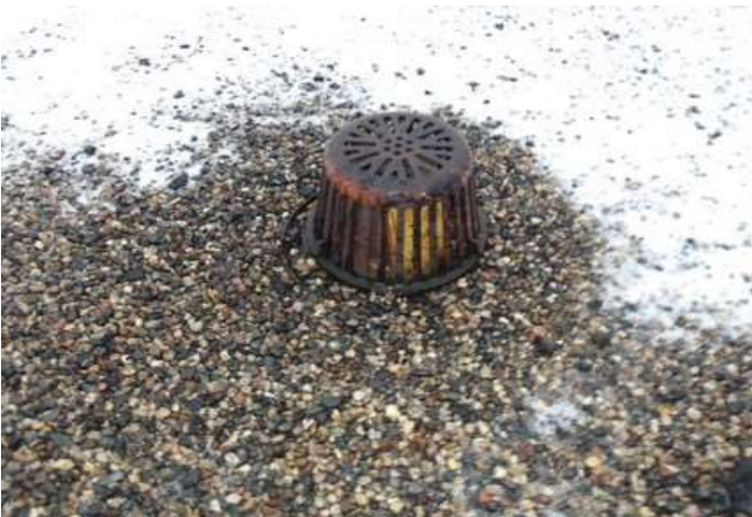
Roof drain penetration
