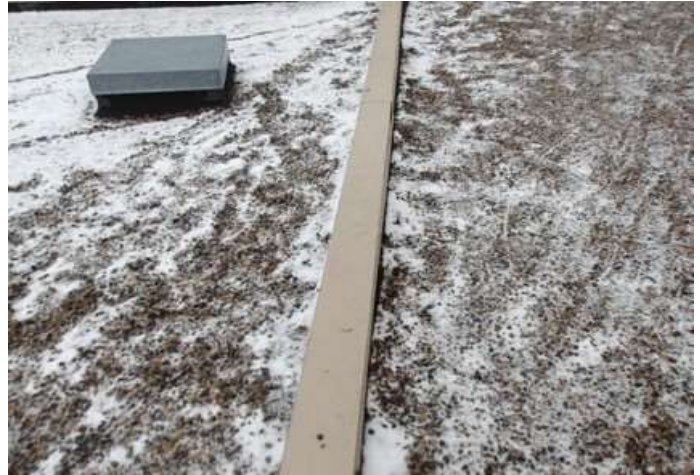
Metal coping between roof sections
