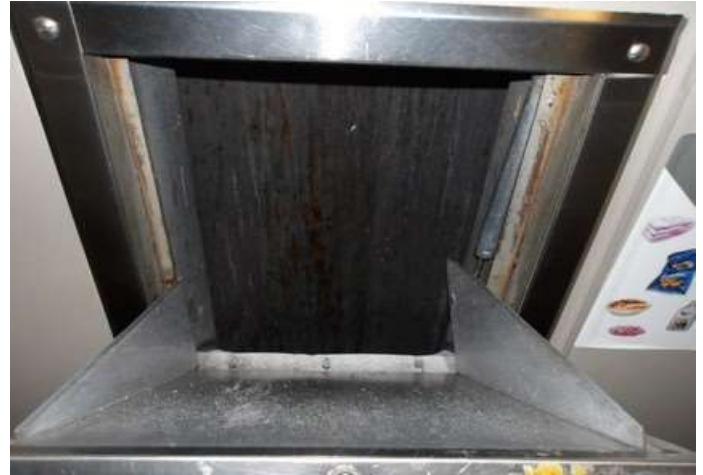
Trash chute liner
