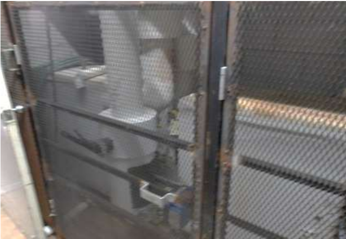
Chilled system heat exchangers (HXs)
