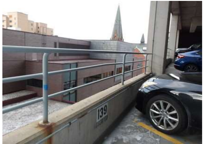
Rust at railing posts
