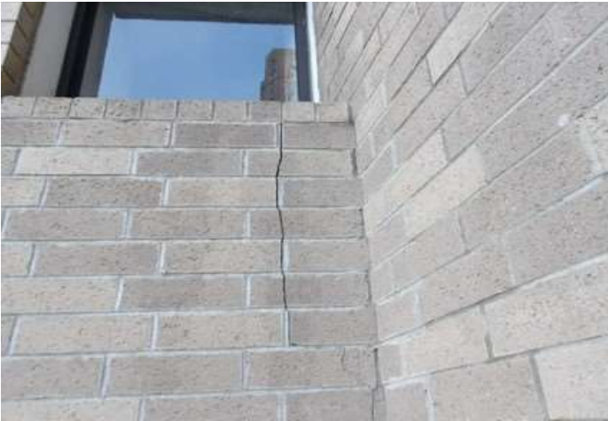
Brick and mortar crack
