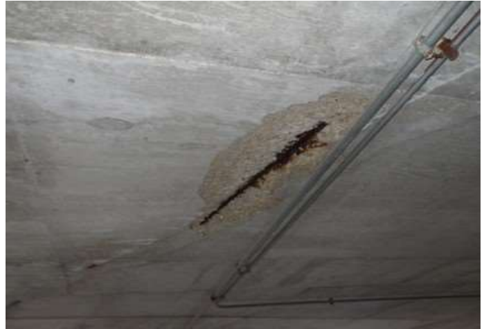
Exposed reinforcing steel with rust
